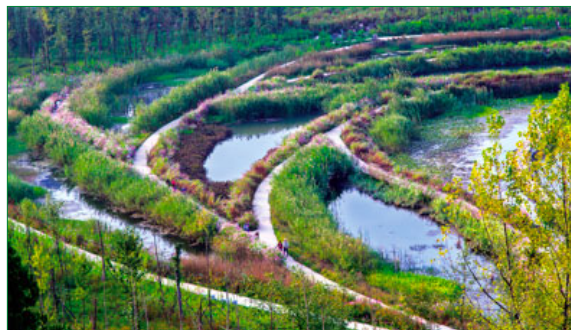
图7 六盘水明湖湿地城市海绵建成实景 Fig.7 Built-up landscape of the Green Sponge System of Minghuo wetland in Liupanshui City
